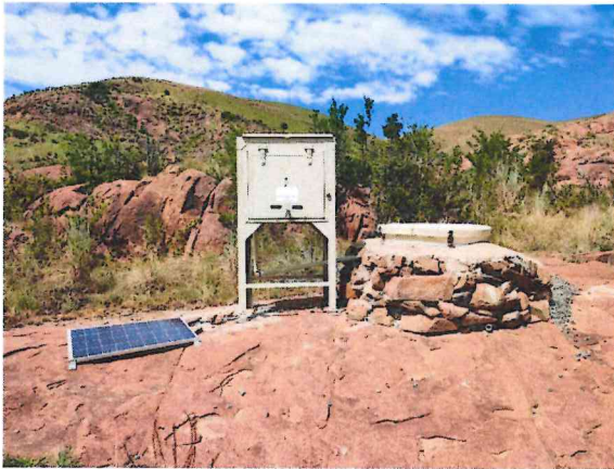
Figure 4: Complete seismic station
